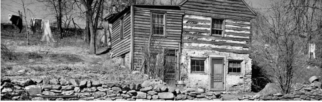
Gover-Matthews Log House, Waterford, VA. HABS VA-775. LOC
